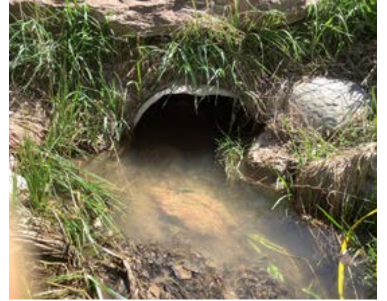
Culvert 20 - 16" culvert directing water under residence driveway.
