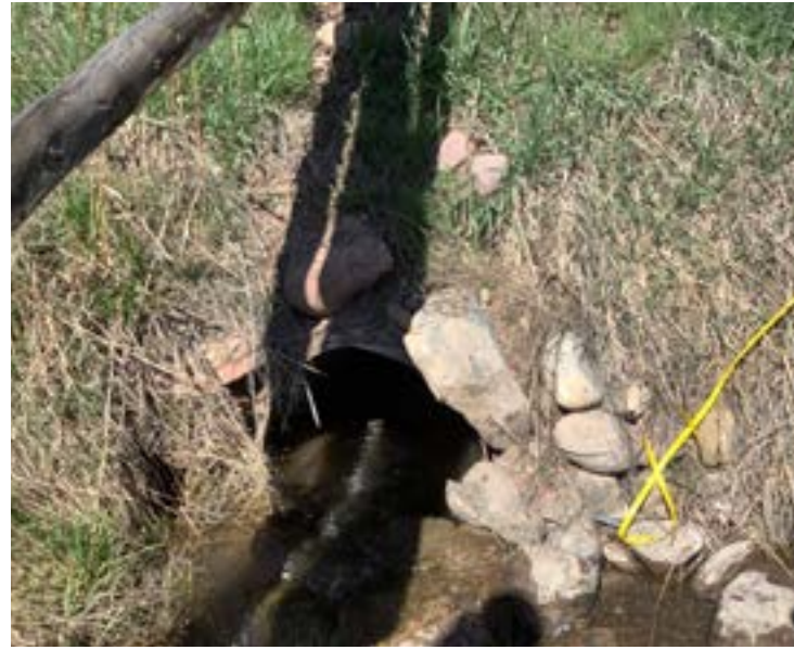
Culvert 10 - 24" Culvert directing water under Driskell Lane.
