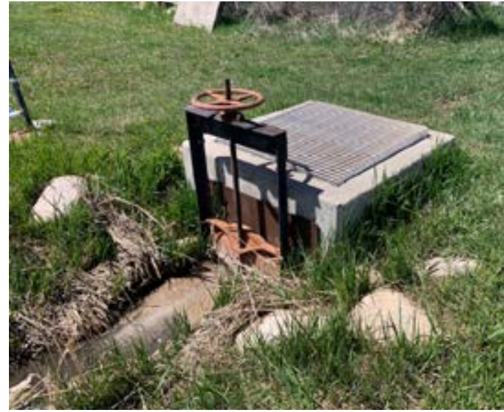
Headgate 3 - Ditch turnout/headgate with concrete box cover. 18" outlet.
