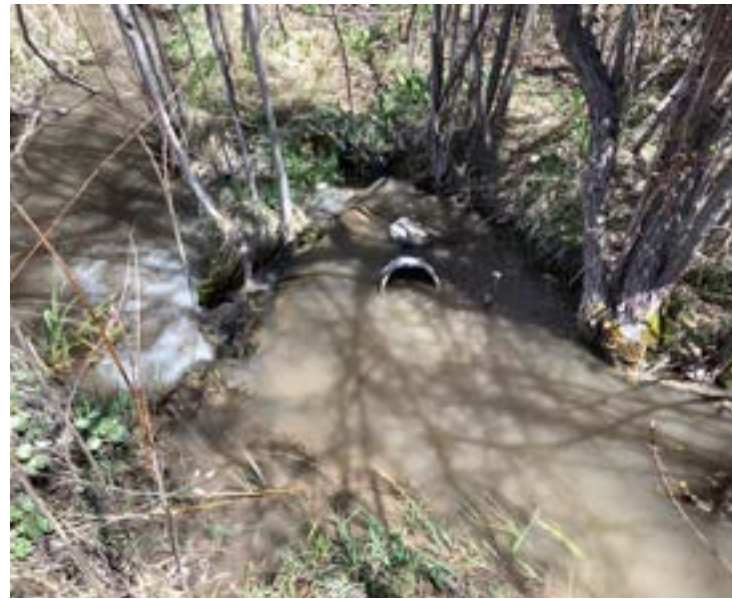
Check Dam 6 - Informal water drop structure/check dam to create pool for pipe intake. Constructed of stacked rocks to control water levels.
