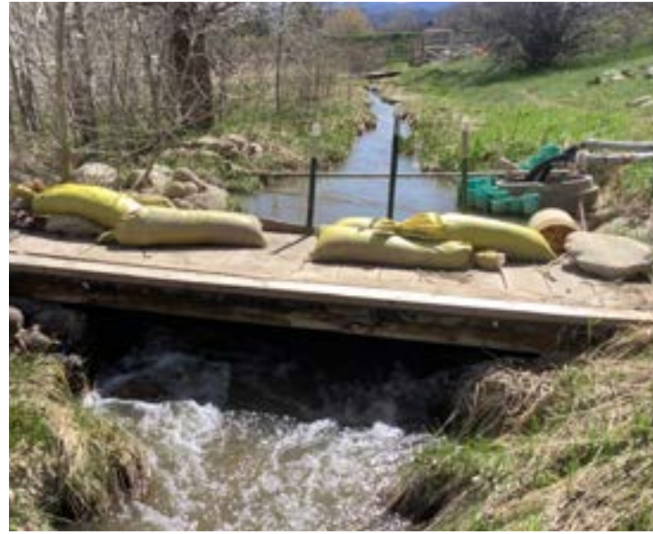
Check Dam 2 - Check dam for pump take out. Constructed of wooden boards, sand bags and T-posts to control water flow. Wooden bridge to access.
