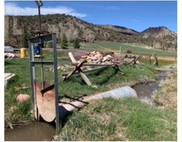
Headgate 4 - Headgate/culvert with 28" corrugated steel culvert.
