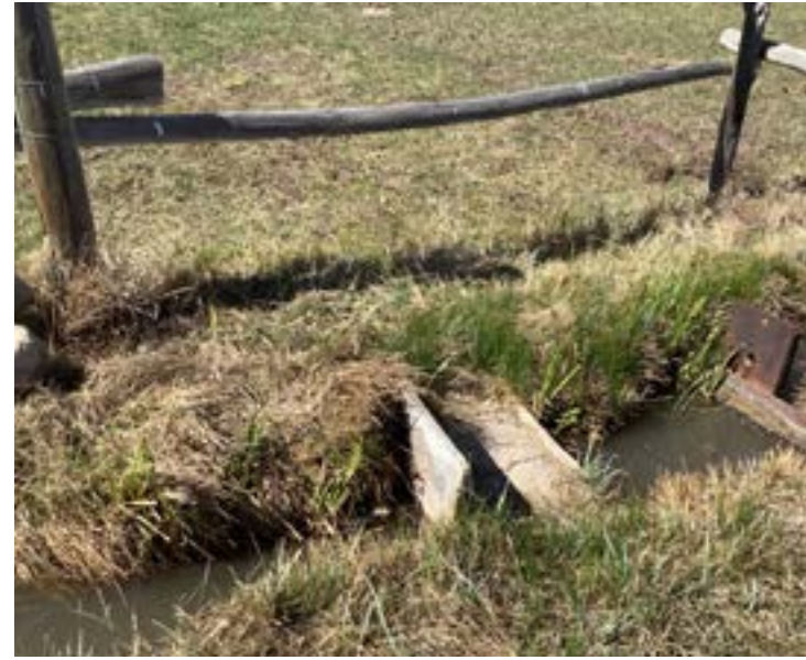
Diversion 3 - Diversion / gate - small concrete structure with wood boards.
