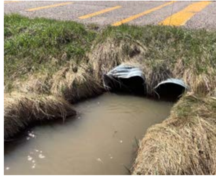
Culvert 11 - Two 24" culverts directing water under Davidson Lane.
