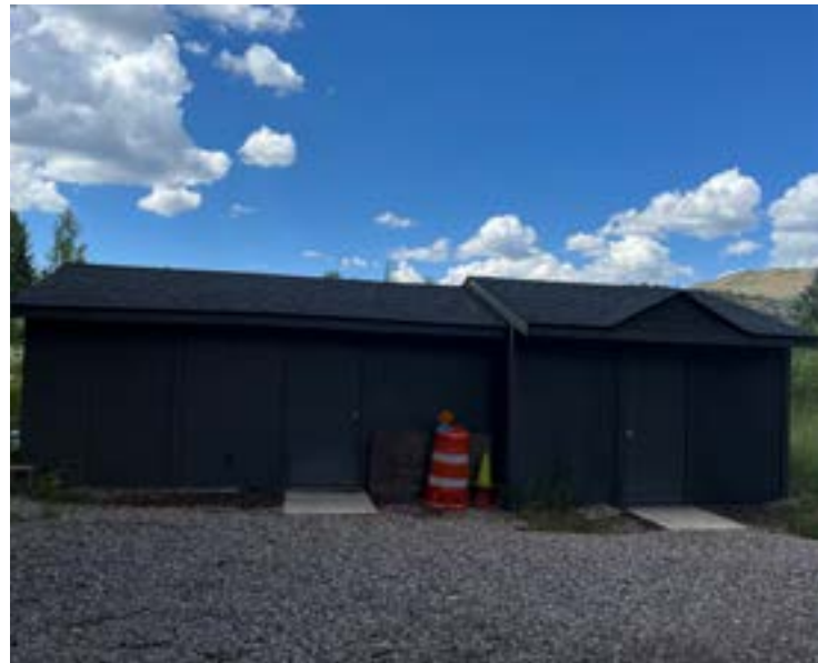
Pump House - View from the south of the front of the pump house with two entry doors.
