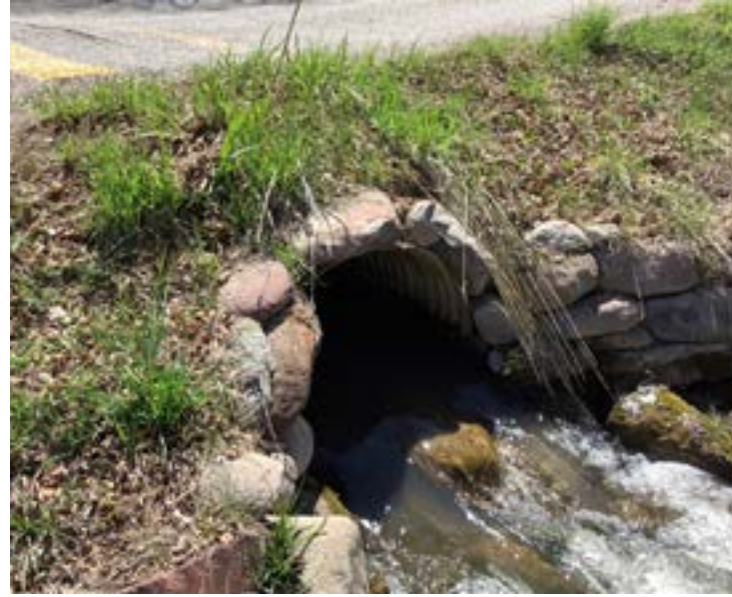
Culvert 18 - 34" culvert directing water under Haystack Lane (Outflow).
