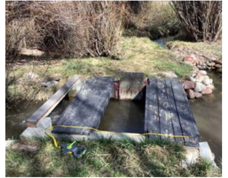
Diversion 4 - Concrete diversion box with gate, 4.5'W x 6.5'L.
