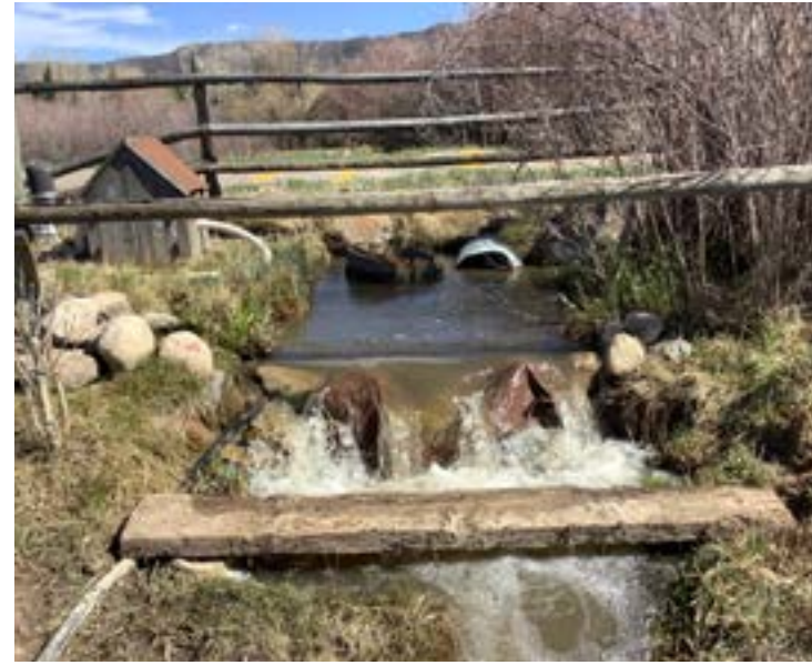
Check Dam 3 - Check dam for pump take out. Constructed of stacked rocks and tarp to control water flow.
