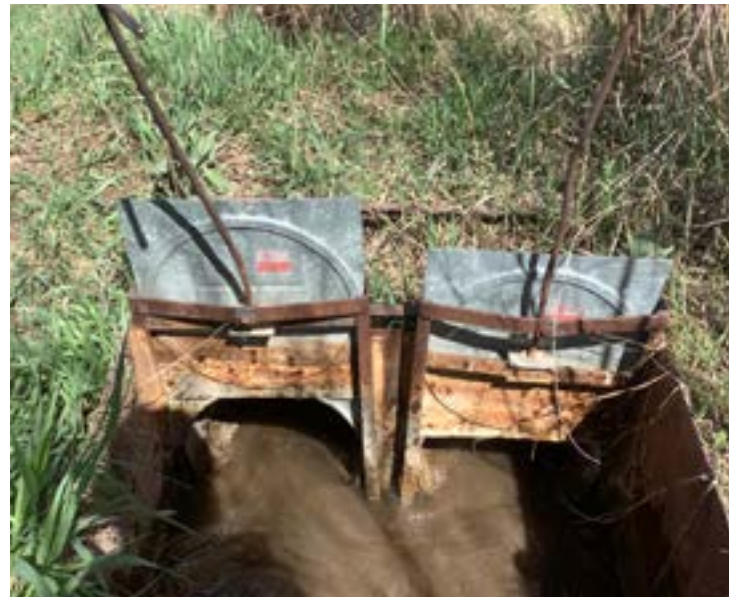
Diversion 14 - Metal diversion box structure with three 12" gates. Two divert Little Elk Creek with one relief inlet from field.
