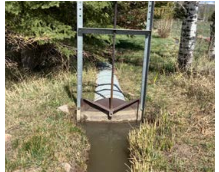
Headgate 8 - Headgate with 26" outlet. Corrugated steel culvert 10' long.
