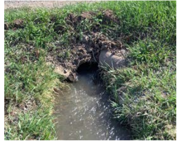
Culvert 12 - Culvert directing water under Haystack Lane (Outflow).
