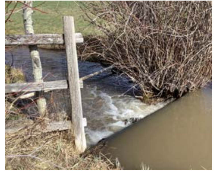
Check Dam 4 - Check dam to maintain water levels for lateral diversions. Approximately 7' across, constructed of rocks with a fence post with tarp draped over to control water levels.
