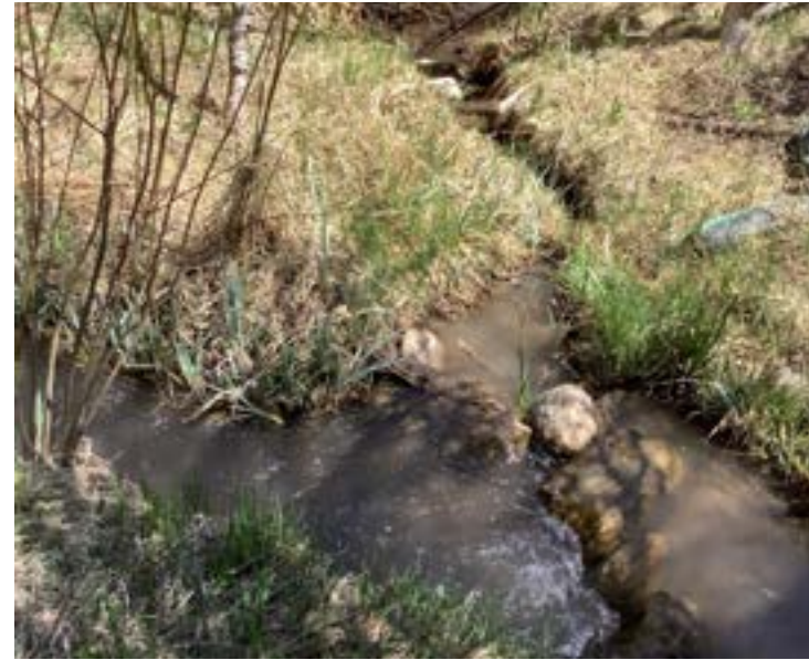
Diversion 11 - Diversion to pond using sand bags and tarp.
