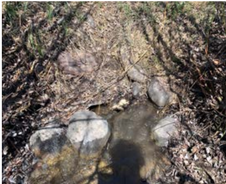
Culvert 5 - 9" PVC culvert, directing water underneath Little Elk Creek.
