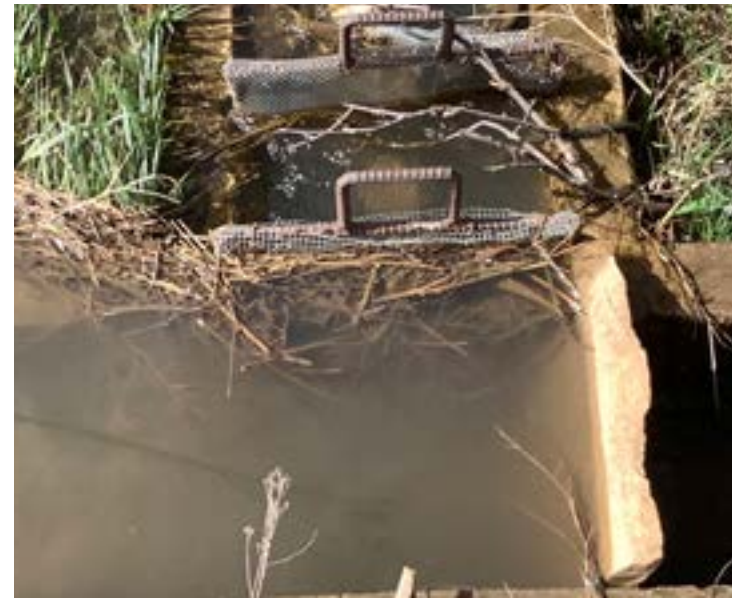
Check Dam 7 - Concrete water control structure with check dam to maintain water heights for pump take out.
