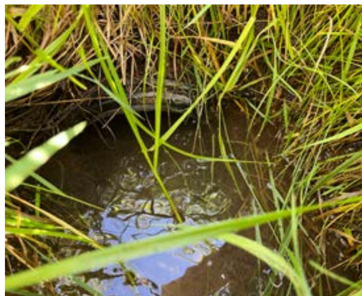
Culvert 22 - 8" culvert in field/side yard for access (Outflow).
