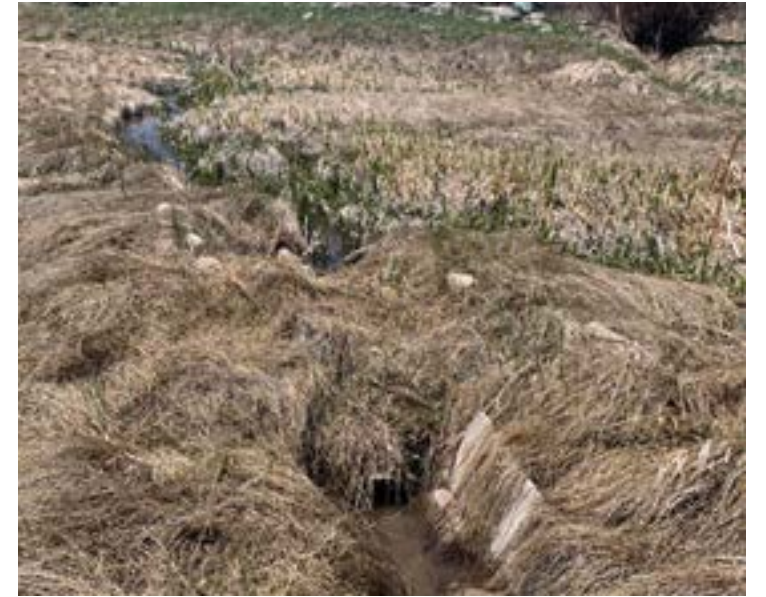
Culvert 4 - 12" culvert at diverting water point of ditch split.
