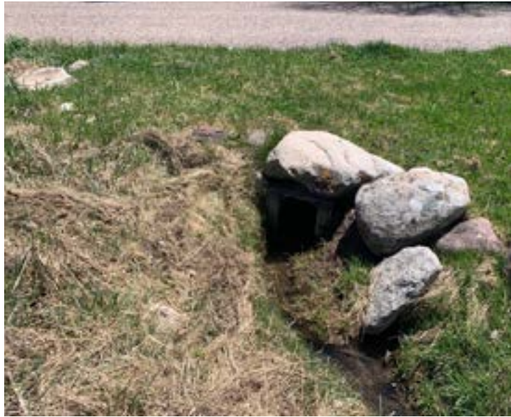
Culvert 1 - 12" culvert, directing lateral under Haystack Lane.
