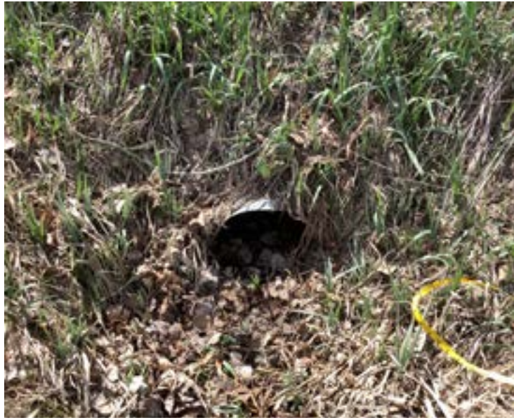
Culvert 9 - 12" culvert directing water under Alexander Ave.
