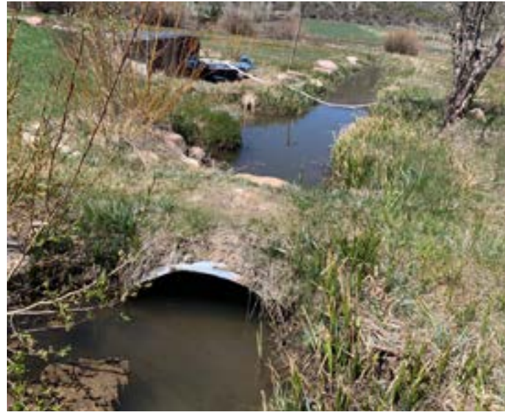
Culvert 6 - 32" culvert for ditch crossing.
