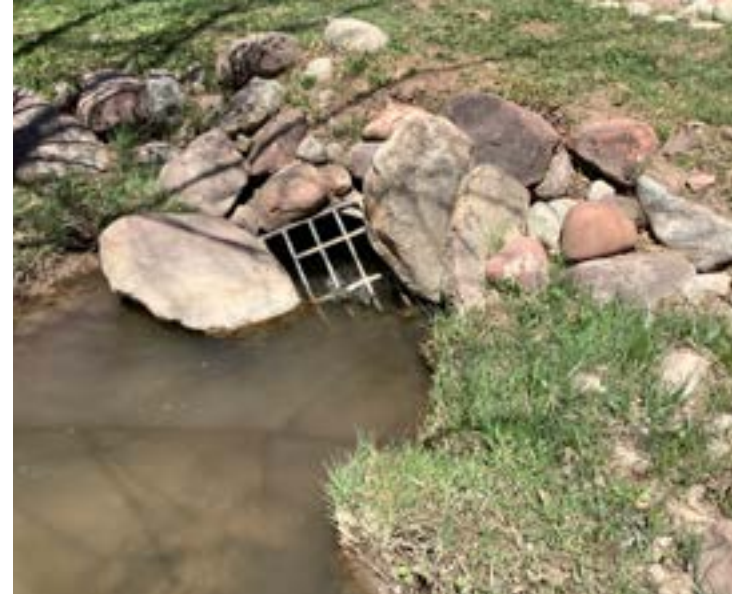
Culvert 19 - 34" culvert with metal grate directing water under Haystack Lane (Inflow).
