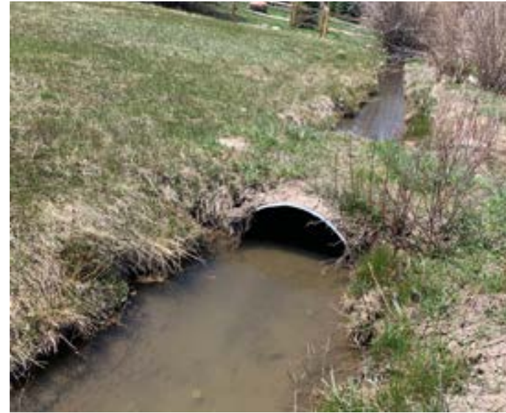
Culvert 7 - 32" culvert for ditch crossing.
