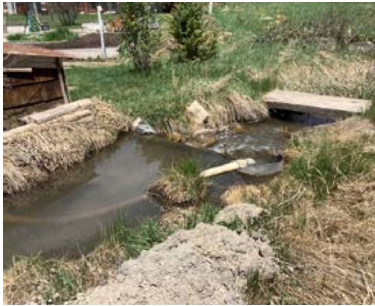
Check Dam 5 - Check dam for pump take out. Approximately 4' across, constructed of metal stakes and boards and tarp to control water levels.
