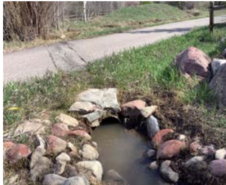
Culvert 14 - 12" culvert directing water under residence driveway (Outflow).
