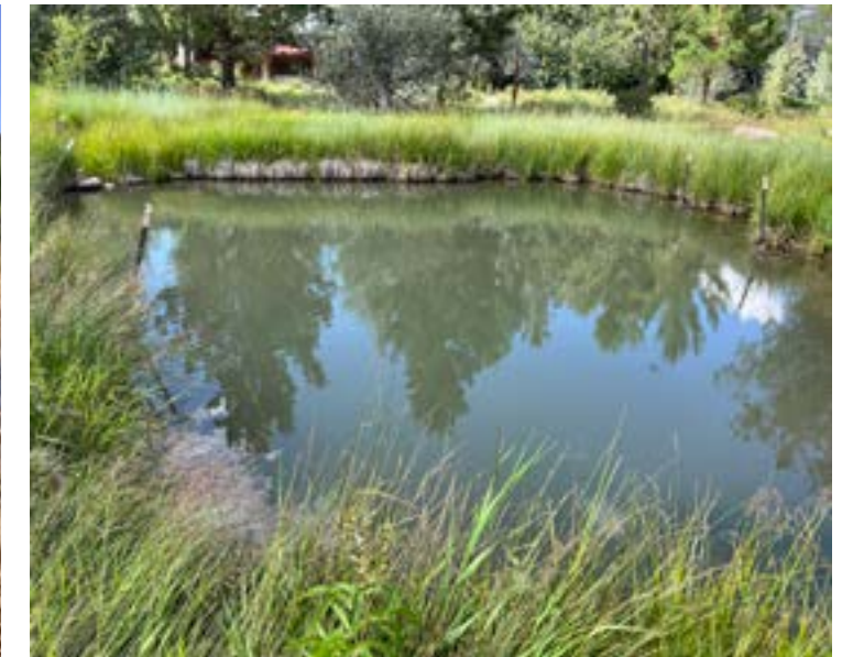
Photo 8 - Upper Catchment Pond - Murky water with low visibility, no aquatic vegetation noted but significant sedimentation buildup from 6-10 inches.
