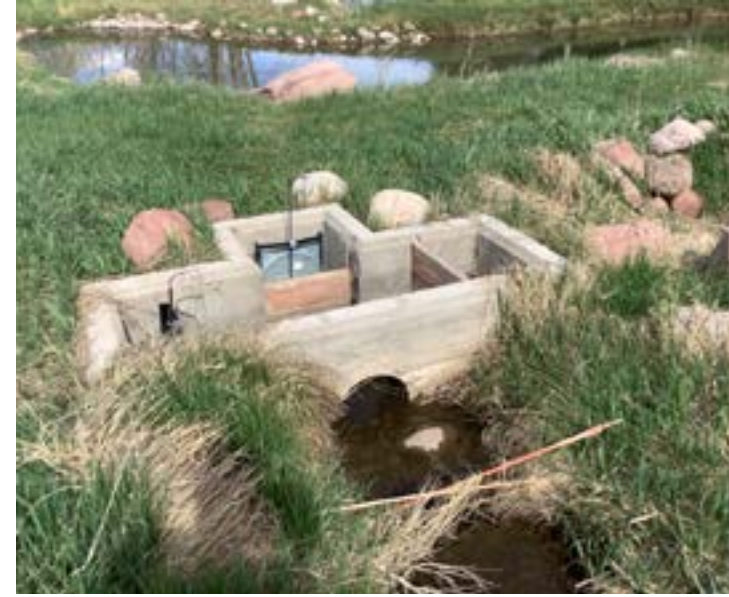
Diversion 19 - Concrete diversion structure with three 1' gates/outlets.
