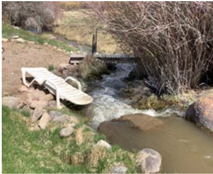
Headgate 5 - Drop feature
