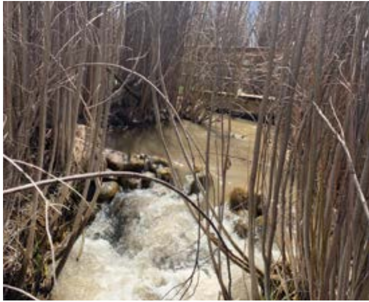
Check Dam 1 - Informal water drop structure/check dam to create pool for pump take-out. Stacked rocks used to control water flow.
