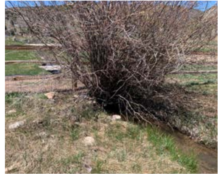
Culvert 8 - 32" culvert for ditch crossing.
