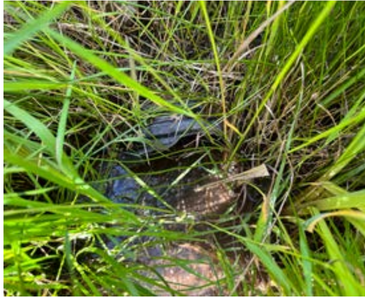
Culvert 21 - 8" culvert in field/side yard for access (Inflow).
