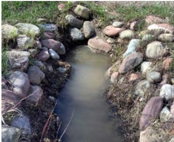
Culvert 13 - Culvert directing water under Haystack Lane (Inflow).
