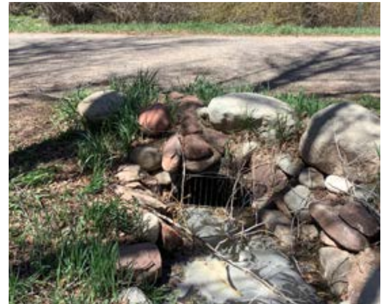
Culvert 16 - 22" culvert with metal grate directing water under Haystack Lane (inflow).
