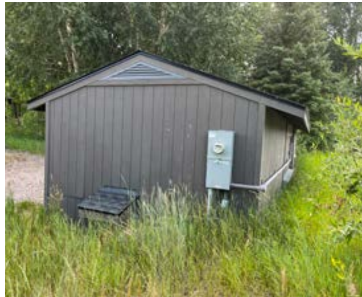
Pump House - View from the east.
