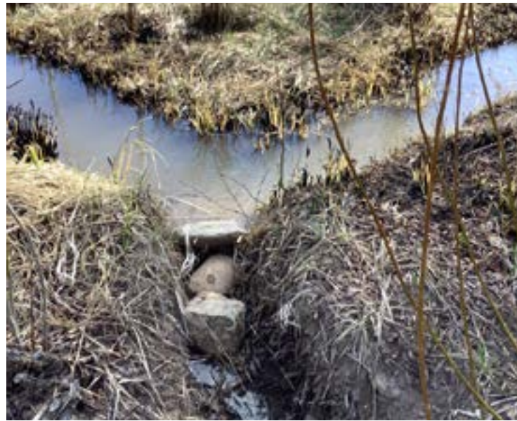
Diversion 5 - Informal turnout with rocks.
