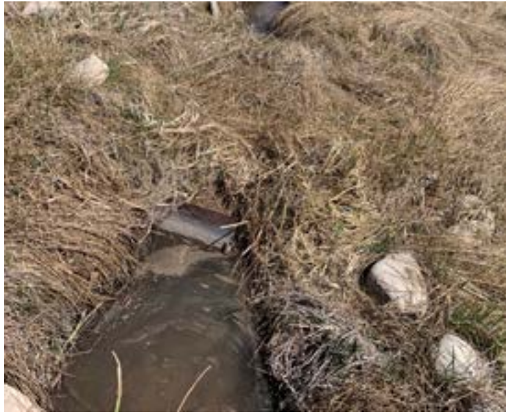
Headgate 1 - Culvert with gate feature.
